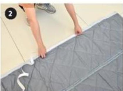
Attach the supplied wide hook tape(A) to the top of the curtain and press firmly. Attach the supplied narrow hook tape(B) to the sides of the curtain and press firmly.
